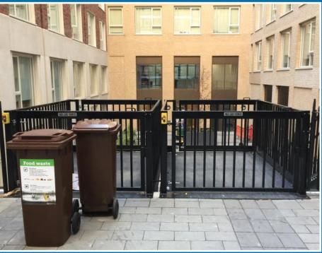
This lift has a raised height of 1400mm and a lifting capacity of 3000Kg. The platform size is 3000mm deep x 2000mm wide. It is equipped with side barriers, interlocked gates, a tread plate platform surface and chainmail mesh skirts. It is controlled from the upper level.
