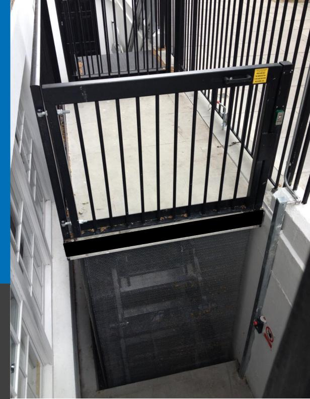
This lift has a raised height of 3000mm and a lifting capacity of 2000Kg. The platform size is 2500mm deep x 2000mm wide. It is equipped with side barriers, interlocked gates, a stone surface platform and chainmail bellow skirts. It is controlled from the lower and upper level.
