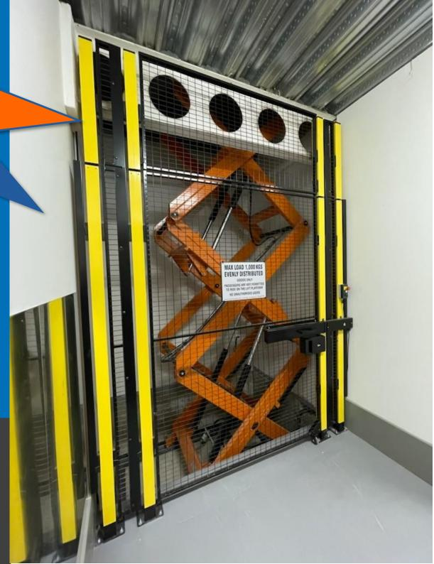
This lift best a raised height of 1600mm and a lifting capacity of 1500Kg. The platform size is 16500mm deep x 1100mm wide. It is equipped with side barriers, interlocked gates, a tread plate platform surface and bellow skirts. It is controlled from the upper and lower level.
